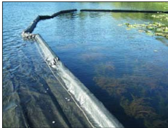
A 100-foot-long turbidity curtain was installed to contain milfoil.
