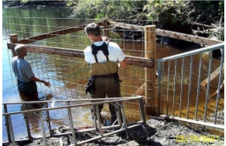
Receiver fence installation
