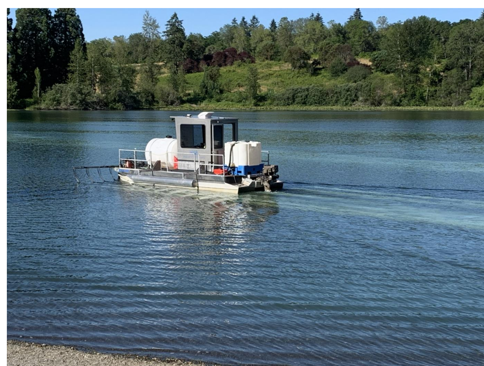
Figure 1. Alum application process at Waughop Lake. The barge drives around the lake spraying alum and buffer together.
